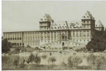
Technical School for Engineers
