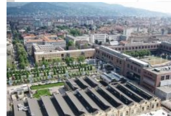
Cittadella Politecnica Campus: site construction opening
