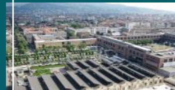
Cittadella Politecnica Campus: site construction opening
