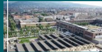
Cittadella Politecnica Campus: site construction opening
